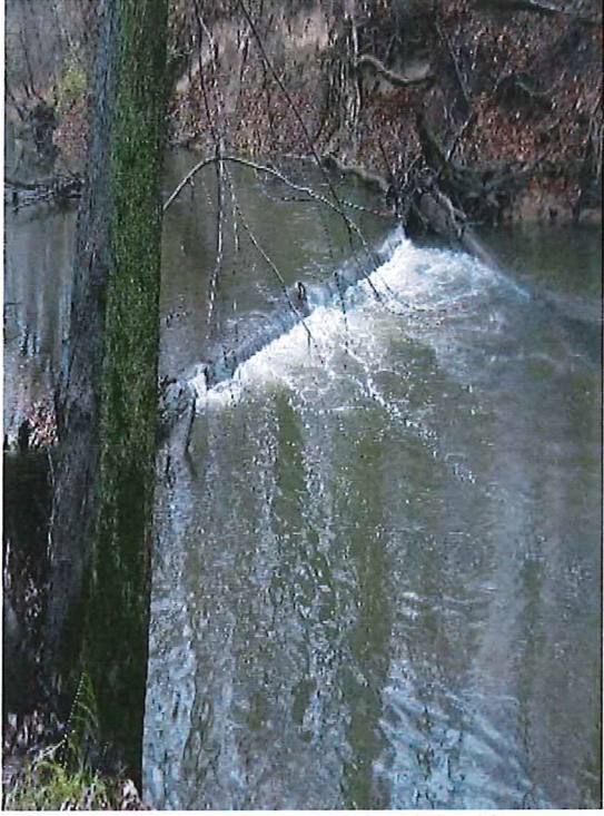
Photo 4 (Section 1 – south bank looking upstream): 8" down tree blocking river flow
