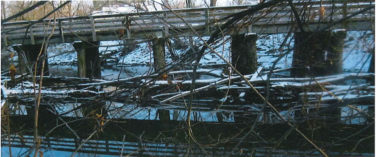
Photo 54 (Section 4 – north bank looking downstream): Piles of branches blocking passage by Kiwanis bridge)
