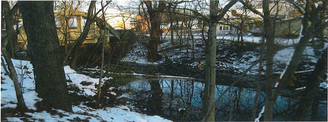
Photo 58 (Section 4 – north bank looking downstream): Downed tree blocking over half the passage through river near Merrick Street Bridge
