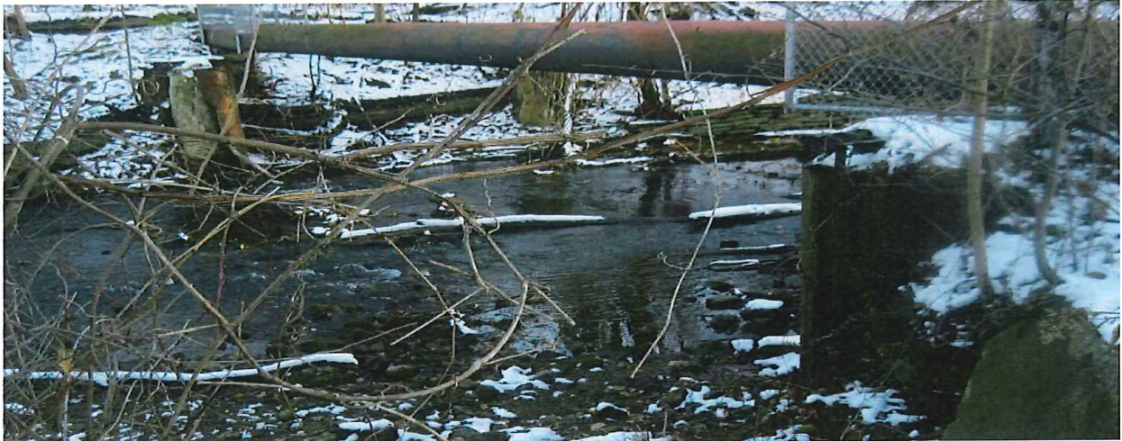
Photo 64 (Section 4 – west bank looking upstream): Tree in middle of river under overhanging pipe
