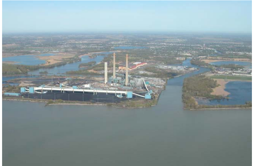
The Monroe DTE Plant with the mouth of River Raisin to the right of the plant (Robert Burns, 2007).
