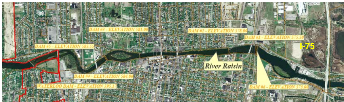
Figure 6-2 Low-Head Dams and Waterloo Dam on the River Raisin in Monroe
